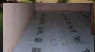
R-10 basement slab insulation
