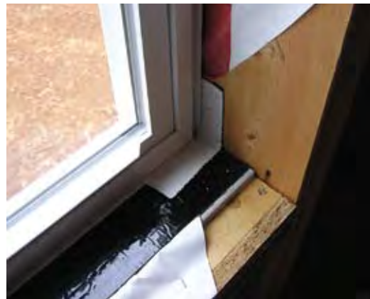
Sloped window sill flashing detail
