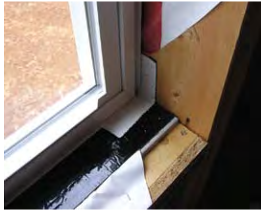
Sloped window sill flashing detail
