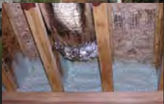
Foundation to deck closed cell foam sealing
